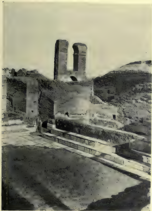
1. Room F, Caldarium , from Southwest.
